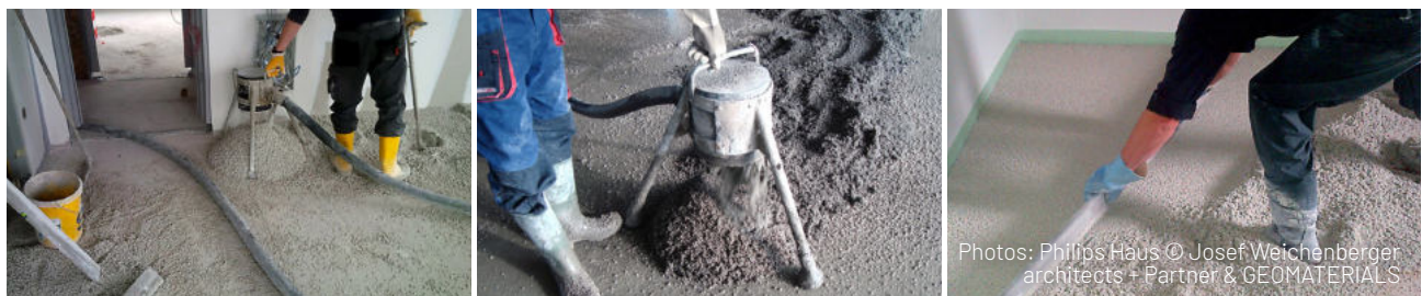
Conveying and application with the screed pump
