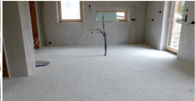
Step 4 - Installation complete All installation cables are encased seamlessly and therefore insulated
