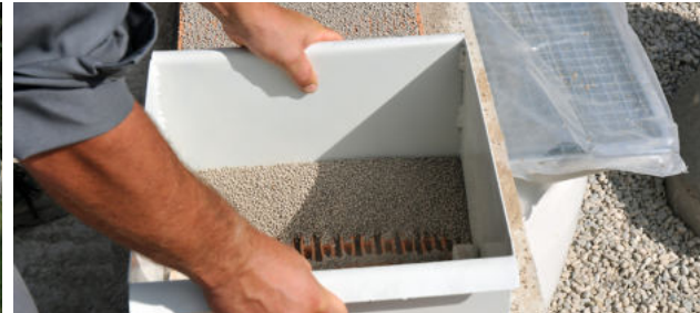
Filling is effortless using a granulate slide that is pushed over the bricks.
