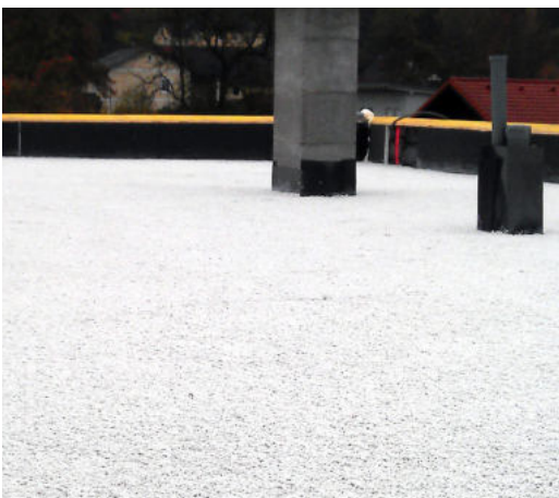
No issues integrating roof penetrations
