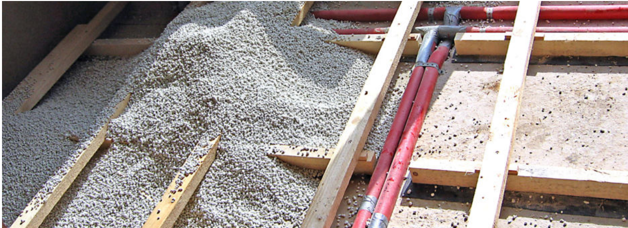
Leveling fill between flooring joists
