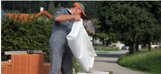
The granules are filled into the brick cavities!
