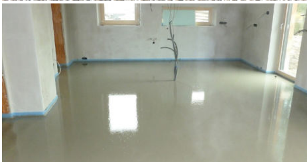
Step 7 - Screed Applied at the desired level in accordance with the reference marker
