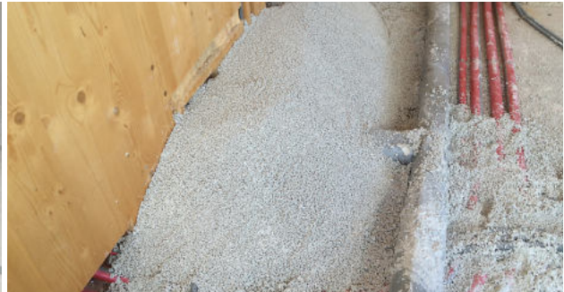
Step 2 GEOMATERIALS Expanded Glass covers all installation cables
